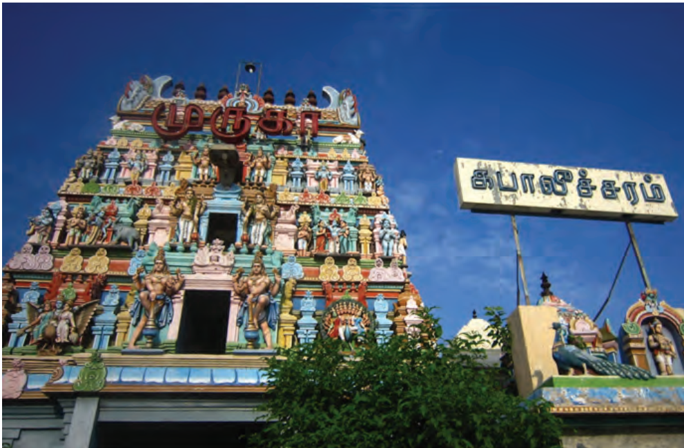
Image 18: A temple dedicated to Tamil god Murugan in Chennai has gopuras or towers covered with deity sculptures typical to Tamil temple architecture.
