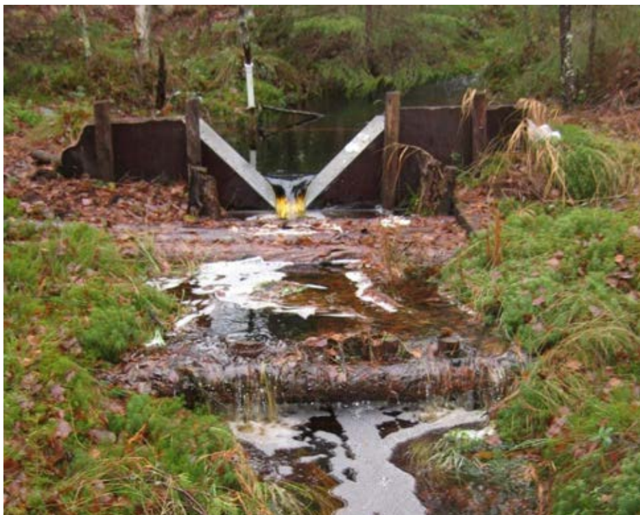
Figure 4. The weir of the outflow ditch. The water samples were collected from the V-notch.
